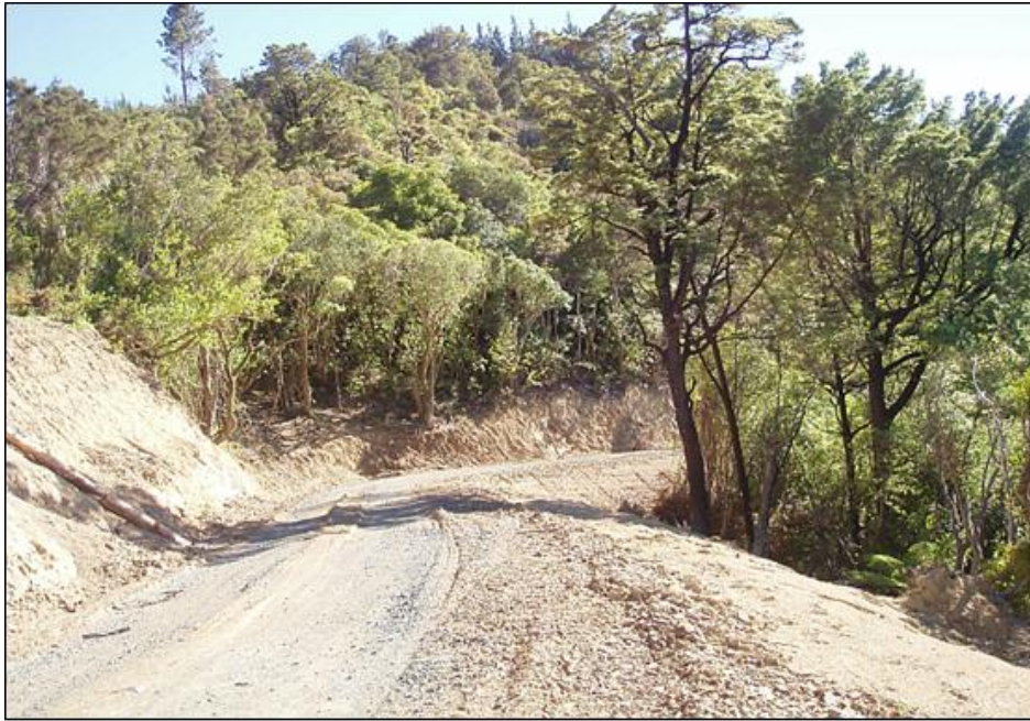
Figure 8: The impacts of bulldozing new haul roads through indigenous vegetation is very significant. Not only does it dissect the native vegetation, thereby creating issues of 'edge' viability, but the spoil from the road is frequently pushed into the bush below, where it can smother the understorey, including threatened plant species and invertebrate communities.
