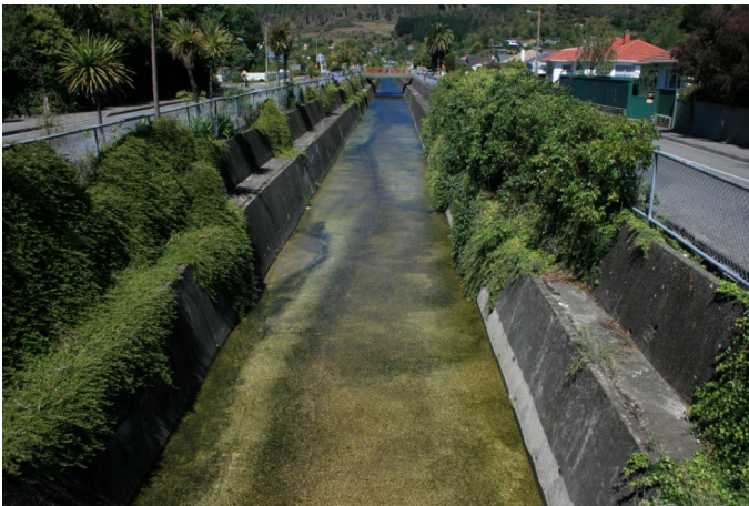
Photograph 6: Brook Stream concrete channel, Nelson
