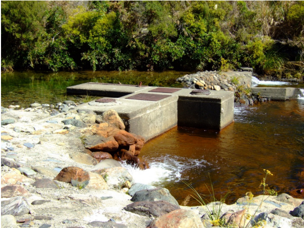
Photograph 5: Intake weir and backfeed discharge, Maitai River
