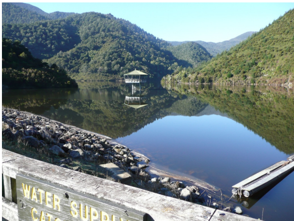
Photograph 1: Maitai Dam, Nelson
