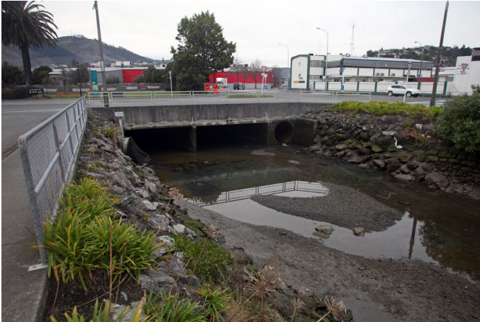
Photograph 7: York Stream culvert, Maitai tributary, Nelson
