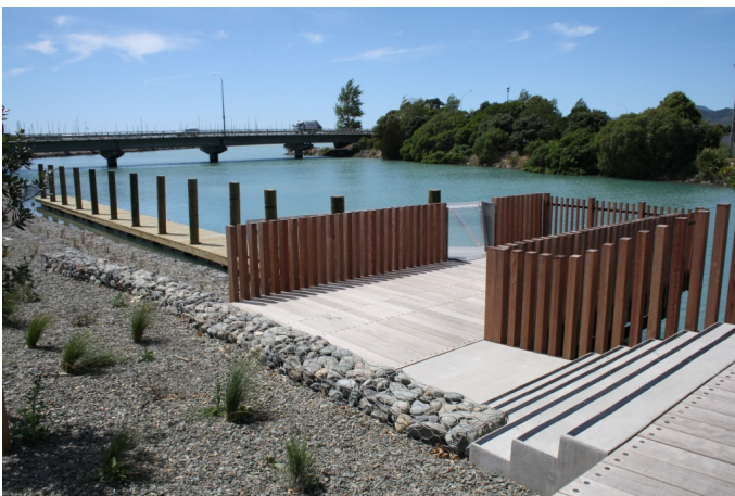
Photograph 8: Maitai Walkway and pontoon development, Nelson
